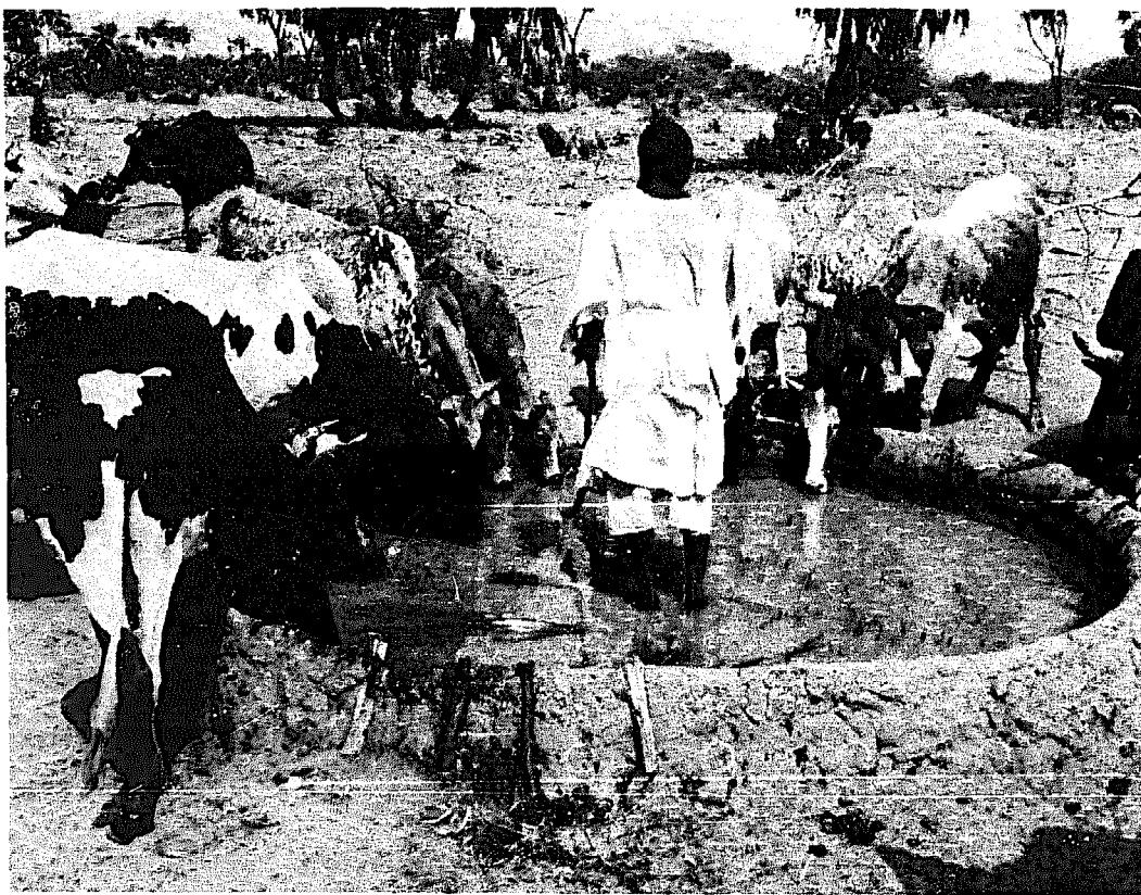
Plate 5.31 A typical shallow drinking trough made from soil.
