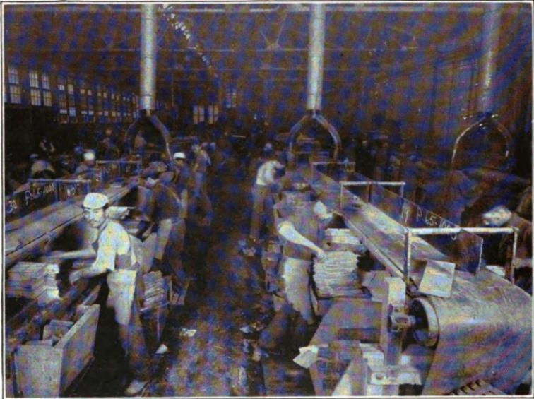
Fig. 40. Pasting Room in the Willard Storage Battery Co. Factory
