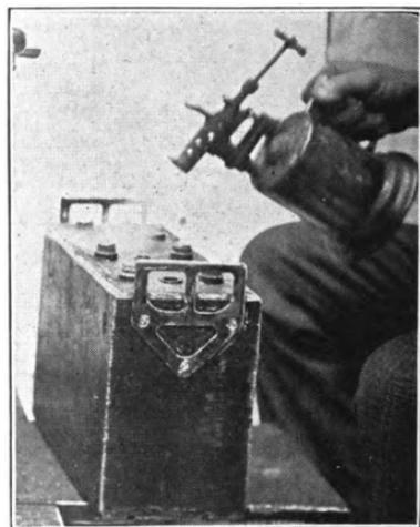
Fig. 103. Heating Compound with Torch
