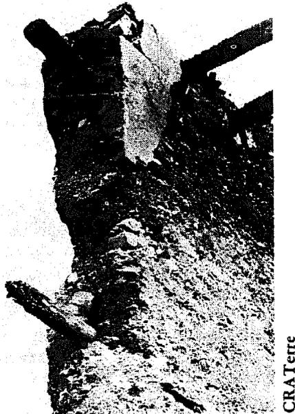
FIGURE 27 : BOIS DE CHAINAGE INCLUS DANS LE MUR DU PISE
