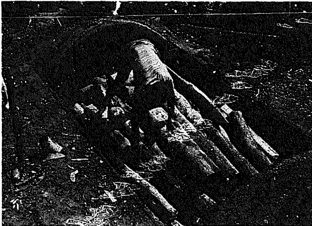
When the kiln is filled to ground level, place the metal sheet nearest the chimney end in position and pack the space underneath with small-diameter wood.
