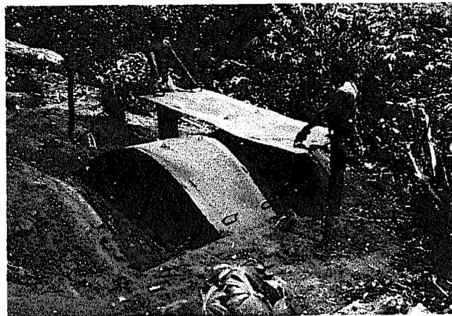
After carbonisation, the contents of the kiln will have shrunk to about two-thirds of the original volume. There is usually a fairly deep hole in the charcoal at the lighting point where the operator can descend to commence unloading into sacks.
