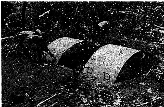
Build up the two end walls with mud and rock to fill in the spaces between ground level and the curved ends of the sheets. Insert the short steam-release tube when building the mud wall at the chimney end of the kiln. The outer edges of the end sheets must overlap the mud walls by at least 10 cm.
