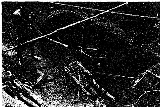
Lay small-to-medium diameter wood across the stringers to form the first layer of the charge.
