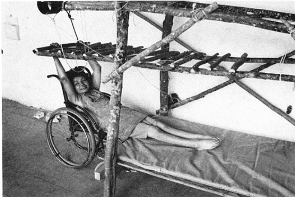
This woman, who has severe spasticity, transfers from wheelchair to bed using tin cans, ropes, and a wood frame over her bed. (Photo: John Fago, PROJIMO.)
