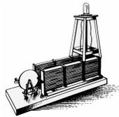
**1832 ~ FARADAY** demonstrates a large version of his first continuous uni-directional electric current generator apparatus, by using the large horseshoe magnet at the **Royal Institution**. (**Note:** This demonstration concerned a homopolar apparatus that was "**not**" acyclic in its nature of operation.)
