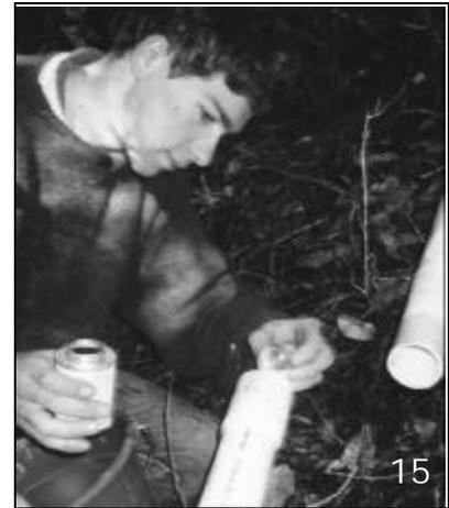
ble, purchase pipe that has a bell at one end, which means the pipe flares out to become the coupler for the next section. This is less expensive than buying uniform pipe that can only be joined by a separate (expensive) coupler.
