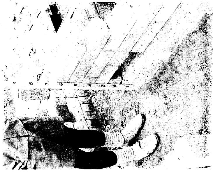
Three 3/8" diameter mild steel rods are placed across the top of the firebox opening to support the front wall.
