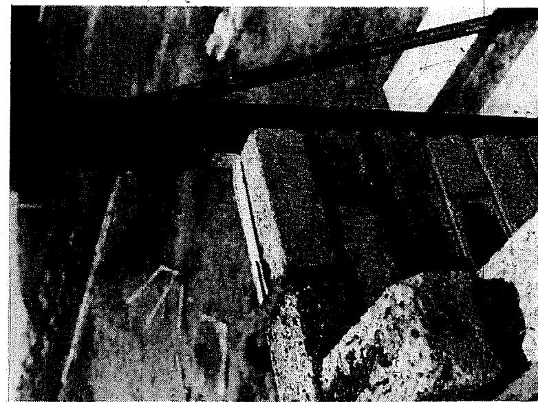
The loading and unloading door of the drier is attached to a wooden frame held in position by hoop iron lugs built into the brickwork at intervals. The top of the frame finishes in line with the top of the brickwork at the front, on which the top plate rests.
