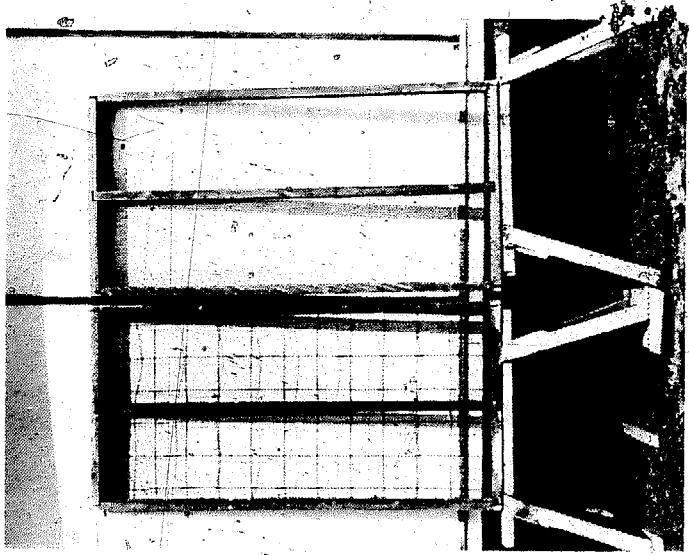
Bolts or mild steel rods are placed in the bed joint of the last course at the back of the drier, thus supporting the pole plate to which the roof sheeting is nailed.
