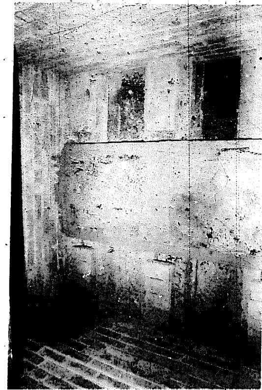
A hot plate of 3/8" mild steel plate is positioned over the hot air chamber on a bed of clay. Clay is packed along the sides and joined to prevent smoke contaminating the copra.
