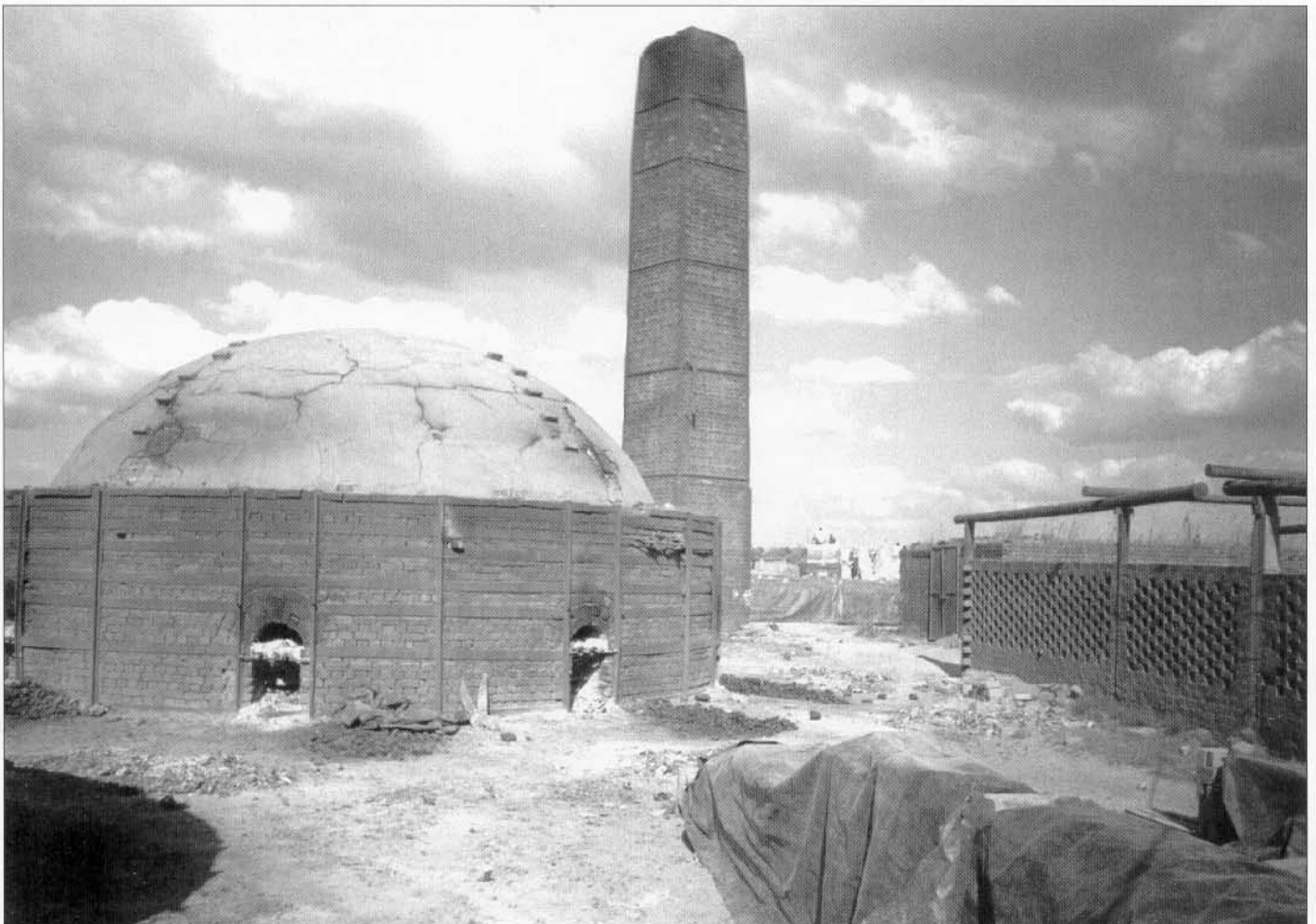
Figure 1 View of an igloo (or beehive) kiln and chimney
