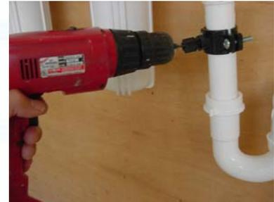
piece of the drain saddle. Now clamp the drain saddle in place 3-5" above the top of the bend in the P Trap. (see photo left) Again, just snug the drain saddle in place. Do not over tighten. Now drill a 1/8 to 1/4 inch hole thru the fitting hole thru one side of the waste pipe. (see photo right) Do not drill into the back side of the waste pipe. Simple wasn't it? Connect enough tubing to the drain saddle to reach the unit 's drain connection.
