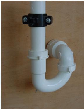
11) The drain saddle. This drain water is the life blood of the system. If the system cannot drain correctly, it will not function for long. The system is self flushing and the drain should never be blocked or restricted. This is really simple. The drain saddle is two plastic parts that clamp over the waste water plumbing of your home. There is small rubber foam washer that needs to be attached to the inside of the connection on one
