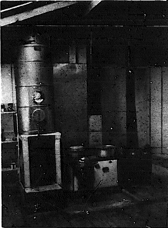
Cooking stove combined with hot water production. The heated water circulates by thermosyphon and water is kept hot in the insulated storage tank. This system has been imported from New Zealand.
