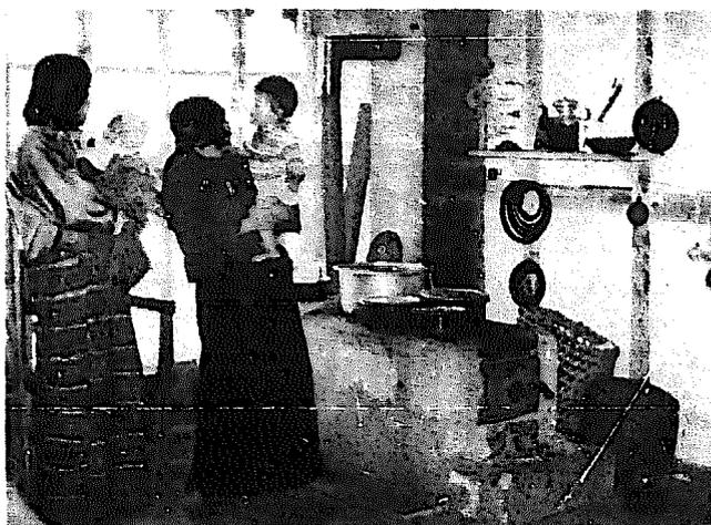
A newly made cooking stove at Bumthang/Bhutan, with cast-iron parts and chimney pipe fitted to masonry chimney.
