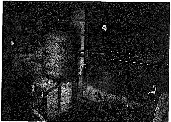
A wood-fired water heater. The insulation around the container keeps the water hot for several hours, (provided the damper is closed after firing)!
