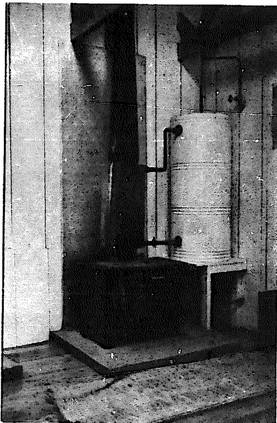
A room-heater combined with hot water production. There is a jacket around the metallic chimney. Note the heat protection on the wooden wall and the solid floor protection (Equipment from New Zealand).
