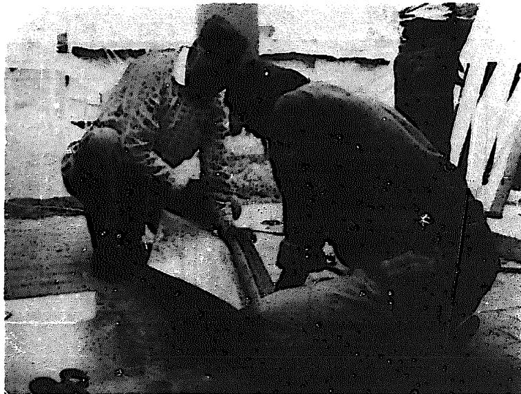
Demonstration of sheet metal pipe manufacturing, using a simple tool made of wood.
