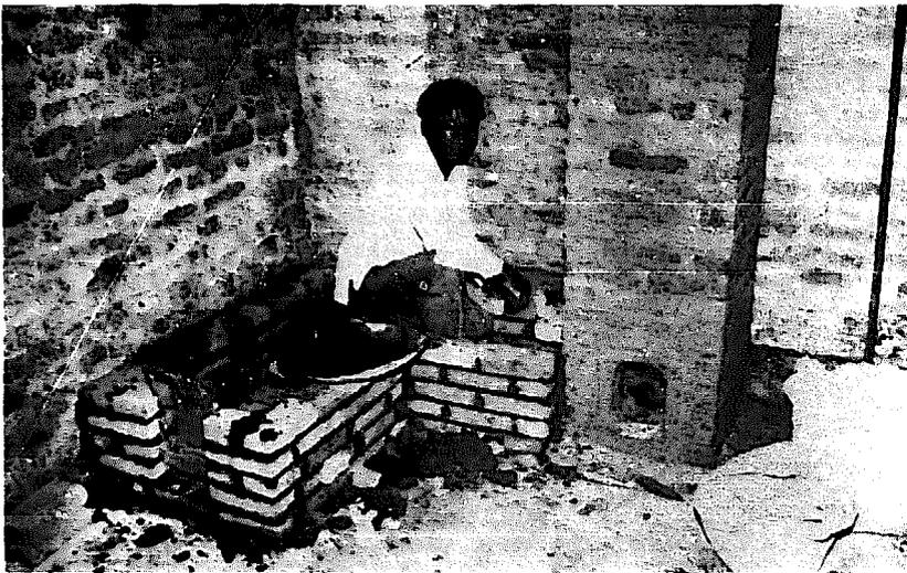
Construction of an improved cooking stove using bricks for the stove-walls and the chimney.
