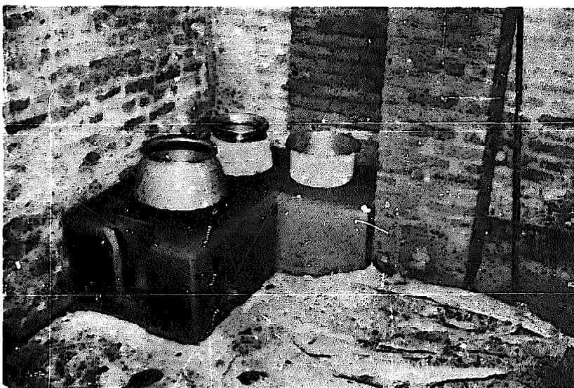
Finished stove, with damper and air flow/ash removal from the side. Note the chimney opening at the bottom for cleaning.
