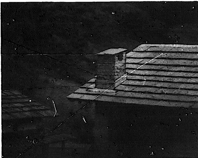
A chimney needs a proper flashing, to protect the house from leakages! This flashing is made of sheet metal by the Mechanical Training Center, Balaju, Kathmandu.
