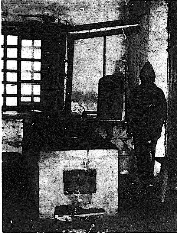
A larger sized cooking range at the Forestry Training Centre in Bumthang. It's cooking capacity is for about 30 trainees, and provides some hot water through a hot water jacket, incorporated in the stove. The hot water container is in the corner.
