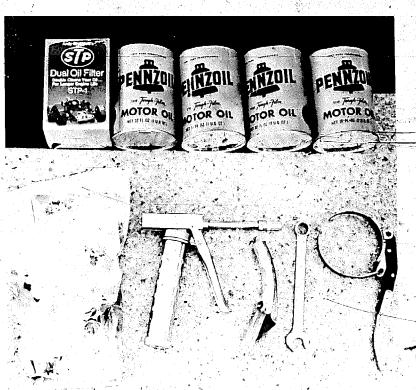
Few-items are required for a complete oil change and lube. Besides oil and a new filter—you need only a small grease gun, an oil pour spout or can opener and small funnel, and a wrench to loosen the drain plug. Filters should be hand tightened, only —but they sometimes get too tight, and a filter wrench is helpful in loosening them.
