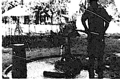
Though the field trials in Tanzania involved only shallow lifts, the combined data from Kenya and Tanzania provides a good basis for judging the performance of the SWN 80 & 81. The pump is very easy to use, with a long pumping handle and the soft pumping action resulting from elastic rising mains.
