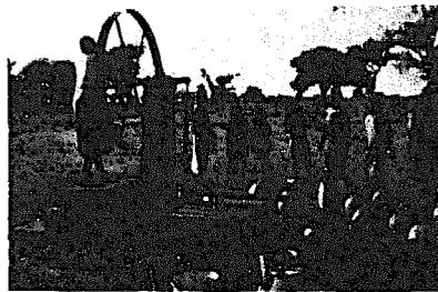
The pumps initially installed in Burkina Faso were of the old design, using a cable as the connection between the plunger and the head assembly and threaded joints for the PVC rising mains. The cables frequently caused poor performance and were eventually replaced with the new arrangement of stainless steel pumprods. Cracks and joint failures occurred in the rising mains until a solvent cement jointing system was introduced.
