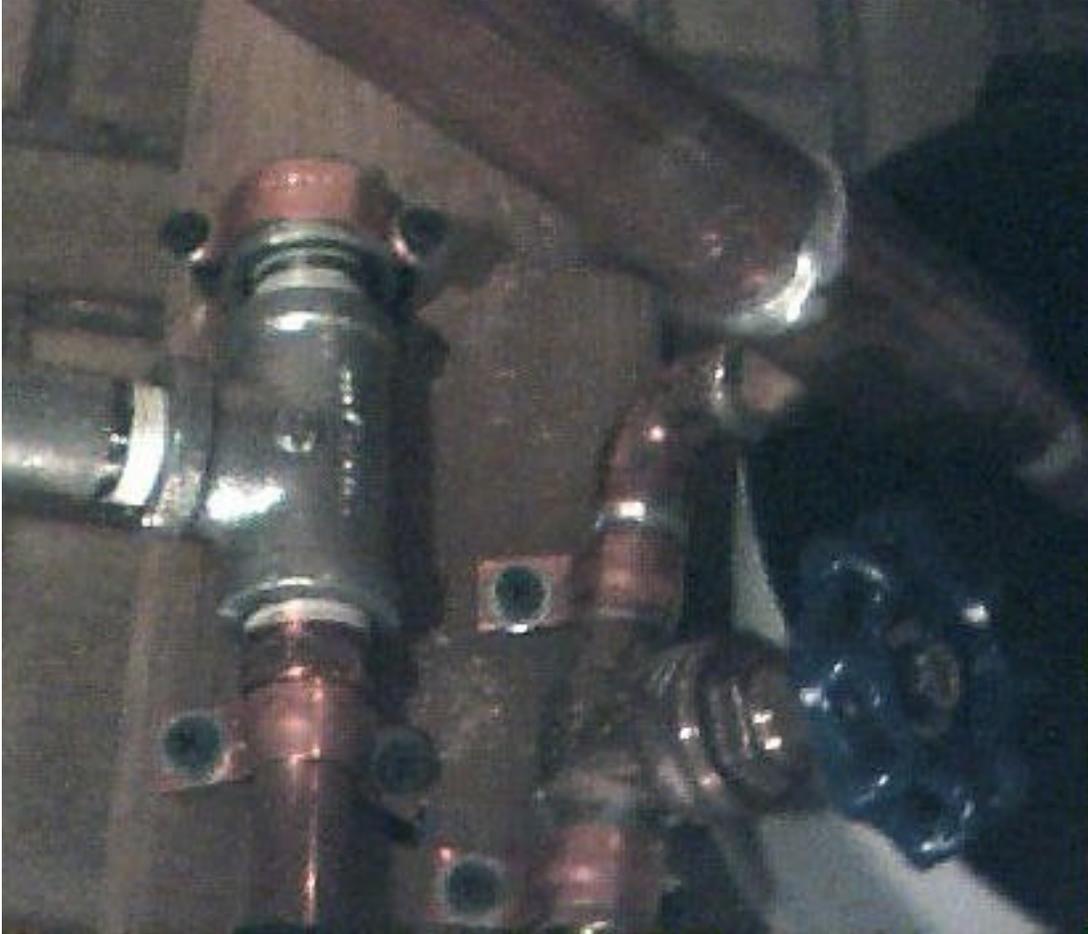
This wooden block (two 2"x4" wood blocks glued together) stabilizes and holds the unit up so that it stands vertically.
