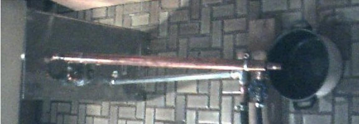
This view is from the back looking forward toward the fire. The flow control for input cooling water and the output flows are all as far as possible from the fire.
