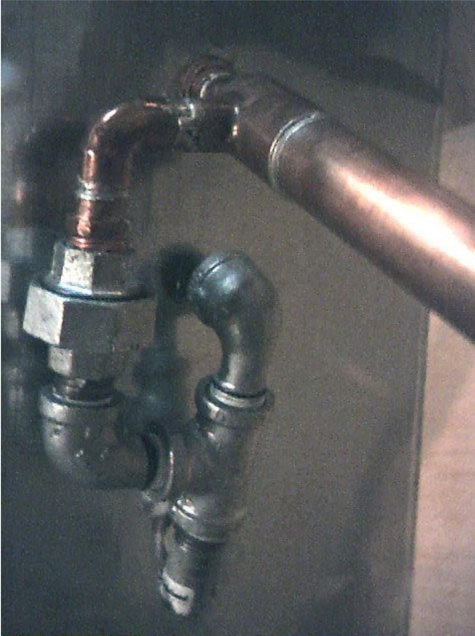
Operates on the same principle as the electric version. Hot water from heat exchanger drops down by gravity and mixes with air to replenish the water level in the lower pipes and to allow the excess to run off as hot water waste.
