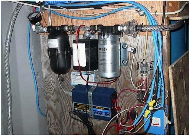
Due to the UV light being turned on only part of the time during pumping of output water, there is a possibility of it taking a number of seconds to warm up. This could allow some pathogens to get by the sterilization chamber. There is also the possibility of contamination getting in the last storage tank. As a result it was decided that the water should pass by a UV light going into and out of this last tank as a safety.
