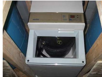
Shown in the center is the pump with it's accumulator that is used to push water through the filters above and the water softener.
