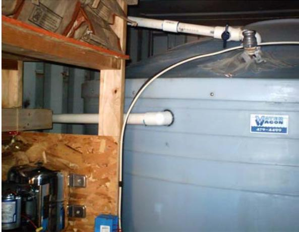
The 1600 gallon container is much taller than the first 55 gallon settling container and expected to fill to a higher level. Thus a ½ inch tank float valve was used in the second tank or the first 55 gallon container to keep it from overflowing. A hose runs between the two.
