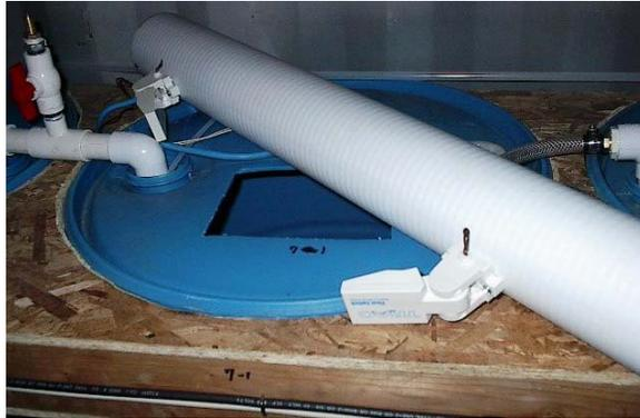
The bilge pump float switch only turns on or closes circuit when the float is up. This is independent of the mounted orientation of the switch. If one puts it in upside down, it will still function the same way. It is open circuited when the float is down.
