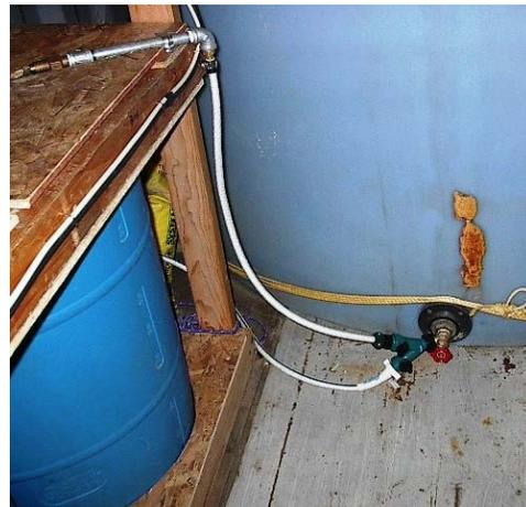
The rest of the holding tanks were made from 55 gallon plastic containers. We had enough of these to double up and use two of these as if the combination were one holding tank. A siphon is used to connect these tanks together so both tanks act as one. To start the siphon going one would pump the air out until one sees water in the clear plastic tubing then shut off the ball valve (as show in the picture).
