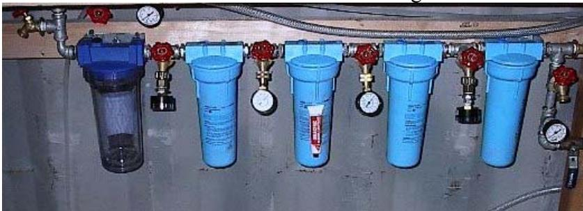
The way the unit is made, one can backwash 1 to 6 filters at a time. Normally we would recommend backwashing only one at a time. However there are times when one will backwash 2 or more at a time to save clean water.
