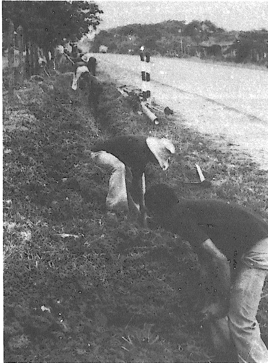
Figure 2.4: Community support in digging trenches for the distribution network, Alto de los Idolos, Colombia
