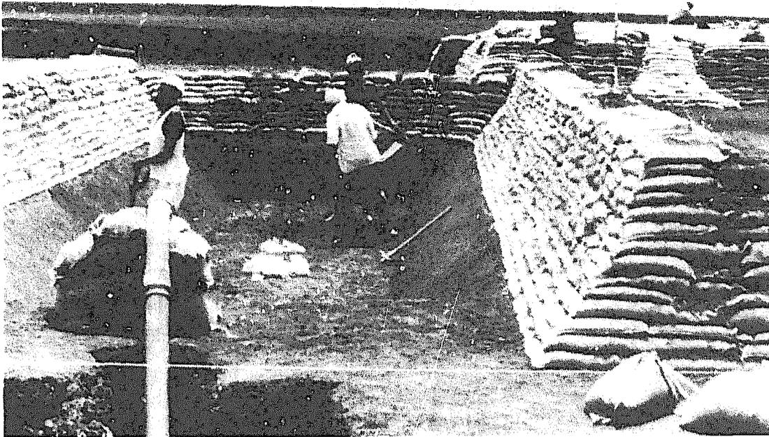
Figure 2.2: Horizontal flow-roughing filter under construction, Fau, Sudan
