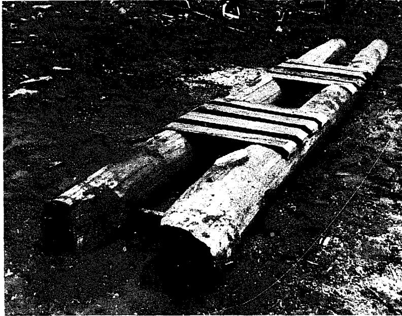
Figure 5. An open-top culvert constructed of wood. Spreaders on the bottom of the logs maintain culvert shape and the 5-cm spaces between the boards prevent water from running down wheel tracks and across the culvert.
