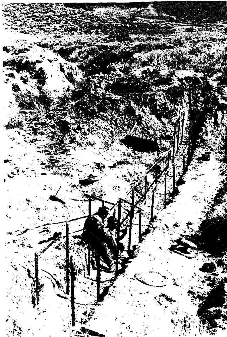
Figure 14. Parallel fences for double-fence dam are being installed. Note the excavations for key, apron, and bank protection, both of the latter to right of the structure.
