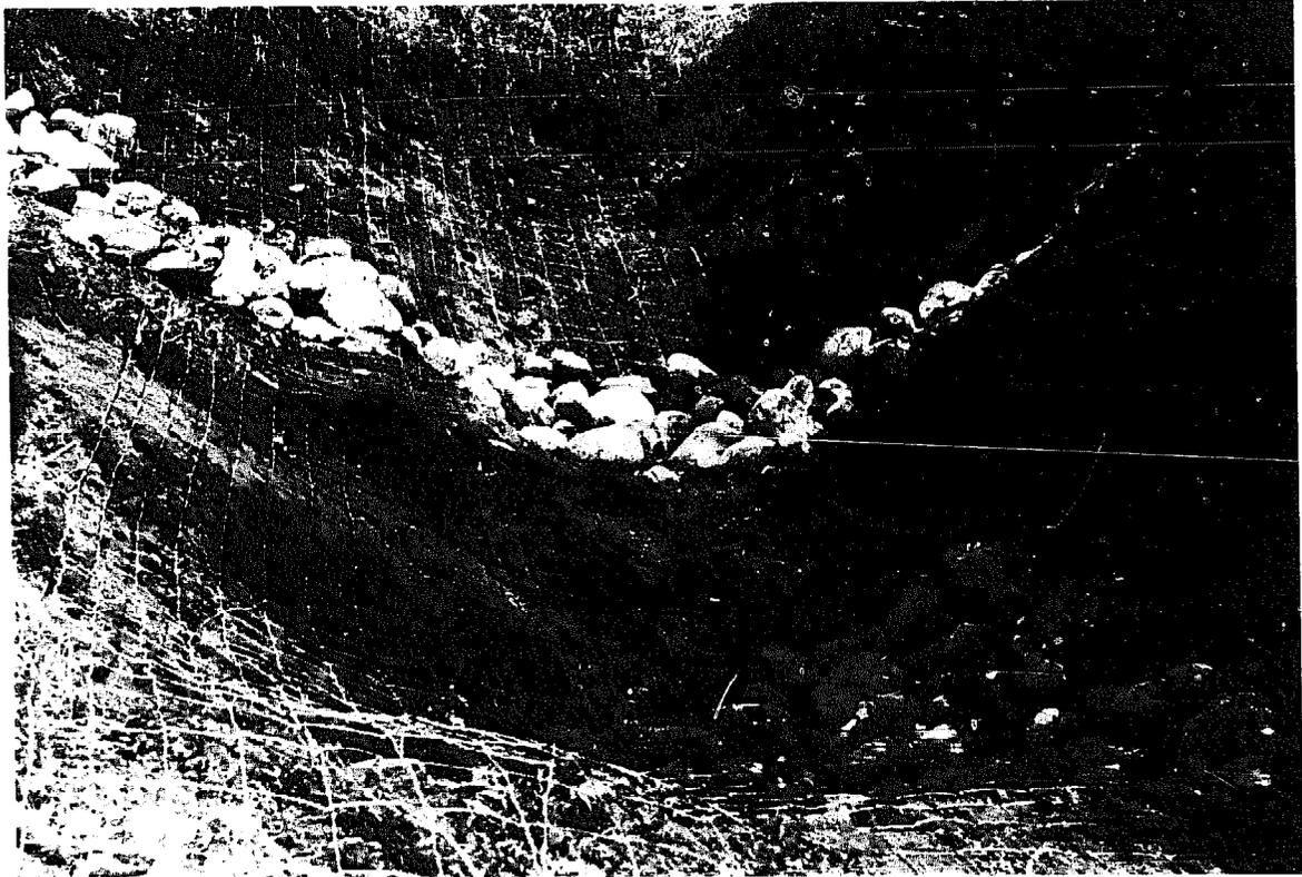
Figure 13. Upstream view of construction site of wire-bound dam. Note that key and apron excavations were filled with rock before wire mesh was placed on the bed and banks. The site is prepared for the construction of the dam proper.
