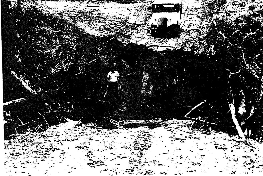
Figure 2 - Earth and log fill crossings such as the one depicted here are potent sources of downstream sedimentation when they become washed out during the wet season.
