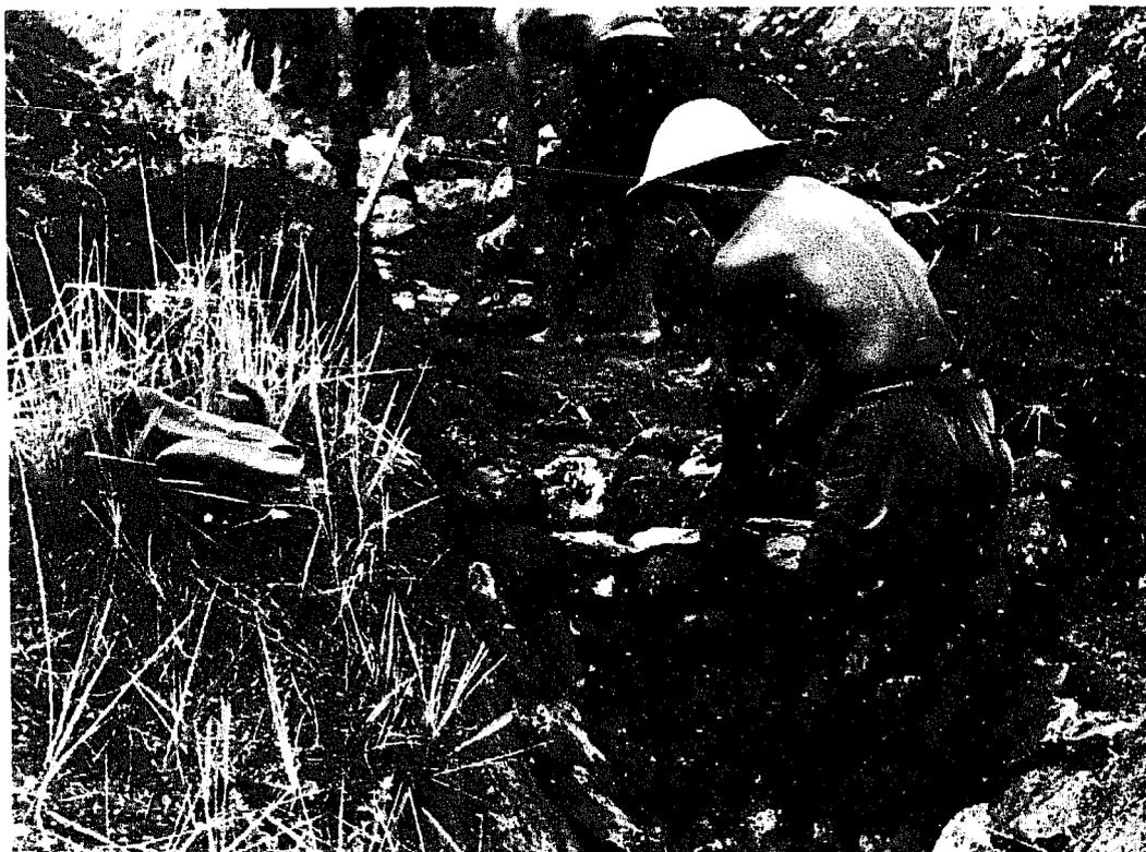
Figure 1. Farmers in Java constructing gully correction works to stop erosion on the Upper Solo River Basin. Part of the efforts on a World Food Programme project (WFP/FAO photograph by J. Bullard)
