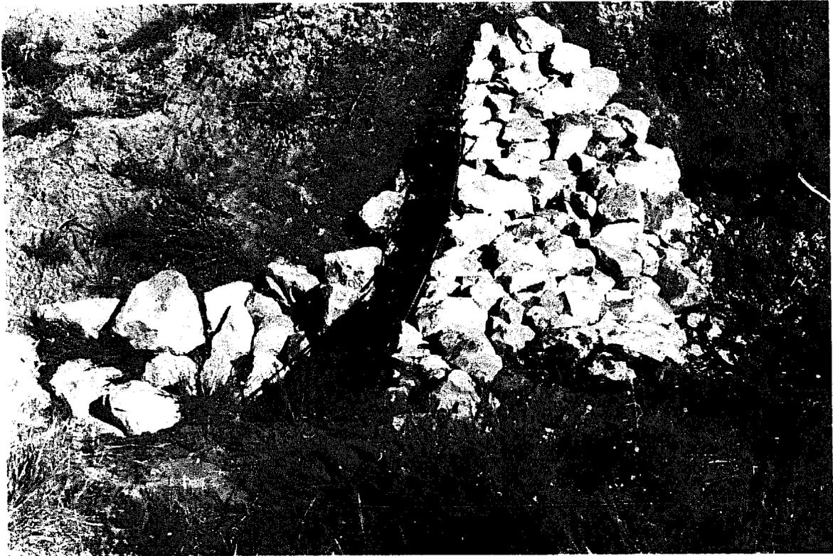
Figure 4. Looking across a single-fence dam. Apron and gully bank protection is to the left of dam crest.
