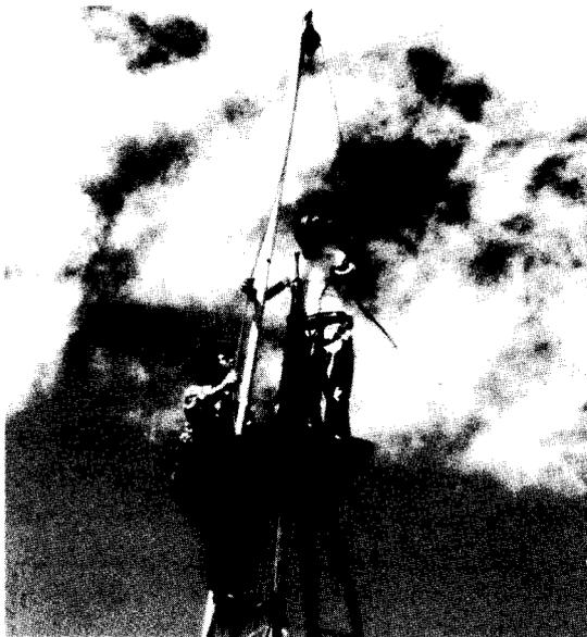
*Figure 5.15. A gin pole in place on the tower.*
