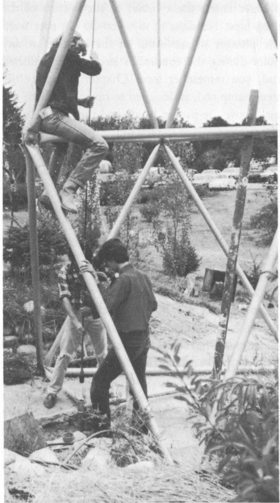
*Figure 5.7. Station an elevated person above the well when lowering the pump rod.*
