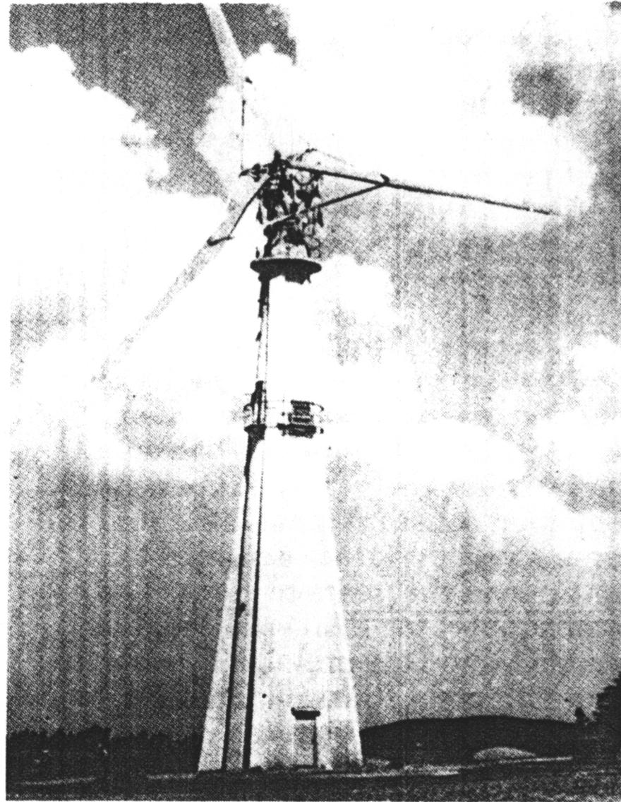
F.L. Smidth "Aeromotors". 1941-43 the company erected 12 2-bladed and 7 3-bladed DC wind turbines with generators of about 60-70 kW.
