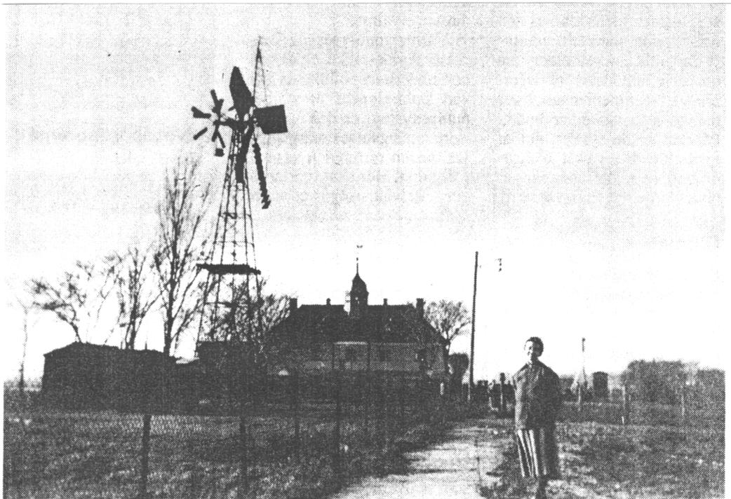
Wind-turbine of Type 1 - 1.5 built 1904. 10 kW DC Generator
